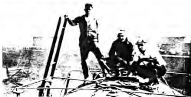
Zenith equipped the first train to use short wave radio. Above is the New York Central antenna installation. G. E. Gustafson (left), the young engineer who built and installed the equipment, has been chief engineer since 1934 and vice president in charge of engineering since 1943. Below is view of caboose before test run.
