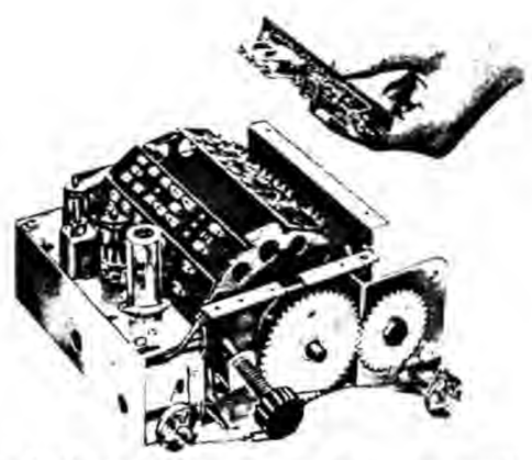
The first Zenith television sets produced in 1948 had provision for UHF reception with addition of tuning strips to advanced turret tuner.
