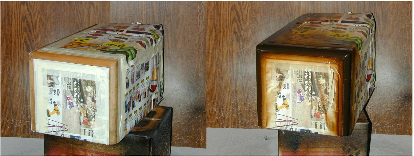
**Fig14: Mask off the cabinet for major trim color-**      **Fig15: Trim with 8 to 10 coats of tinted lacquer.**
