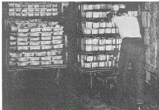
Each lead mold is flipped on its side and air hammers are used to tap the radio cabinet out of the lead mold, by hammering on the edges of the cabinet, directly through the soft lead. Usually, the cabinet comes out of the mold unscathed; sometimes it is broken up in the process. The picture (below, left) shows the typical Catalin pieces (square rods) being hammered out of their lead mold. The lead mold is always damaged in the process, and is
