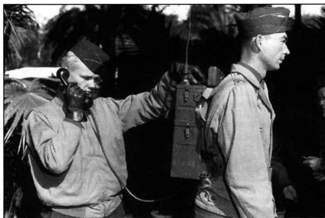
The well-liked "Walkie-Talkie," SCR-300, a good FM transceiver built by several manufacturers.
